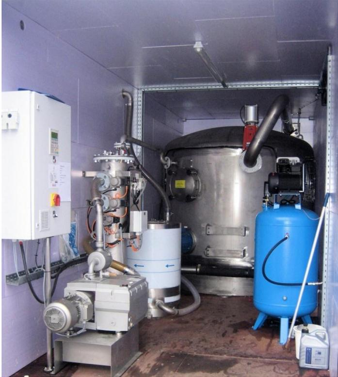
Figure 3: External container containing food waste tank and pump
